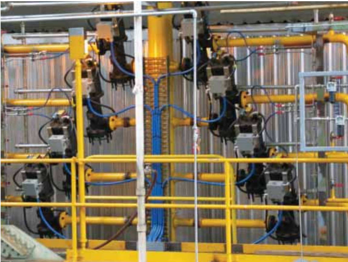
Shown are eight T4300F (3 inch) Skotch Trifecta gas valve systems replacing the need for twenty-four independently actuated valves. Considerable installation time and space are reduced.
