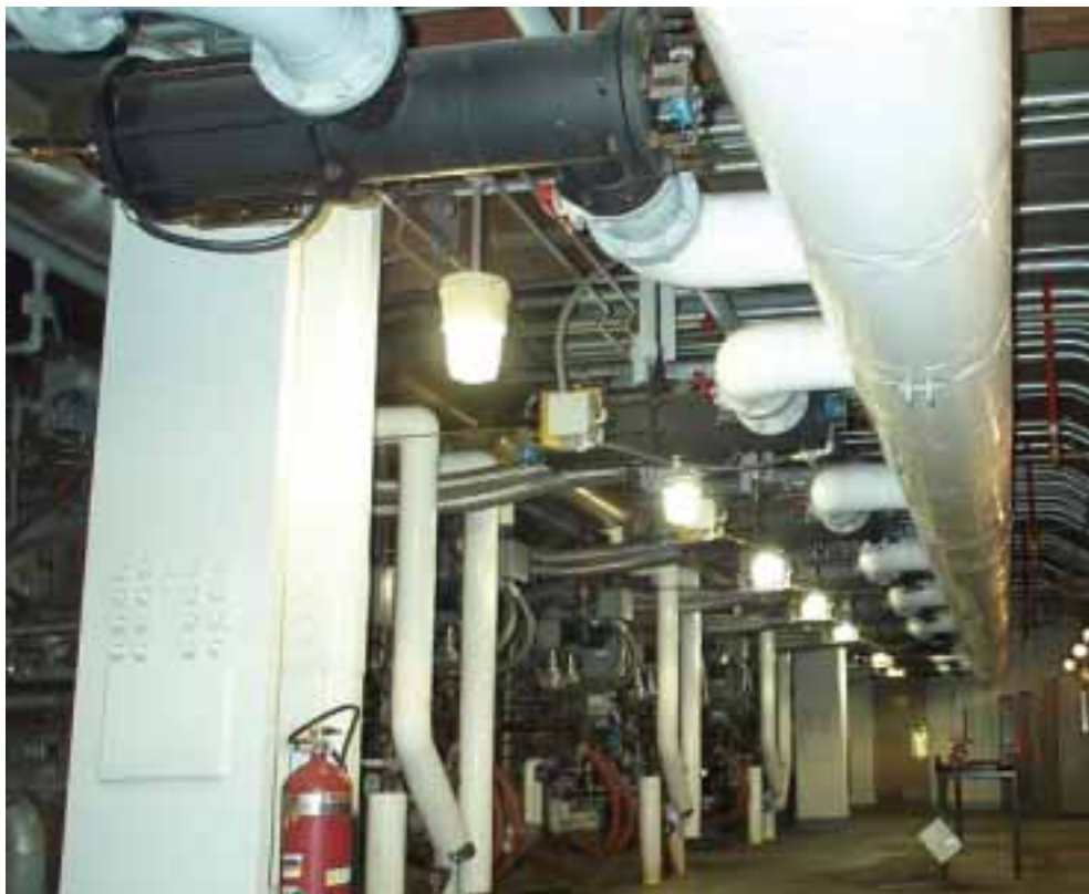
T4600F (6 inch) Skotch Trifecta gas valves are installed above the burner level in the horizontal position which reduces burner front clutter.
